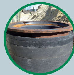
Ø600 well raised with riser rings and floating frame
